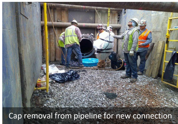
Excavation with trench boxes for safety
